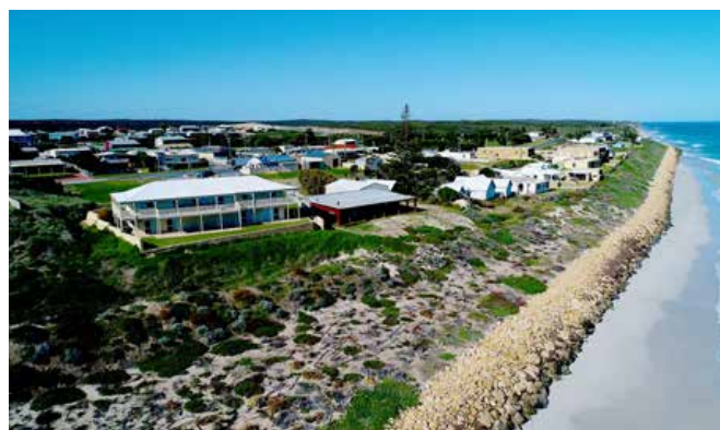
Coastal seawall in the Shire of Gingin
