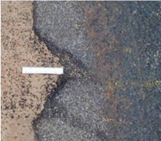
Figure 9.2: Photos of onsite edge break width measurement
