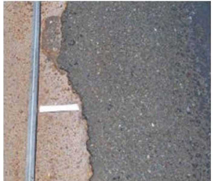
Figure 9.2: Photos of onsite edge break width measurement
