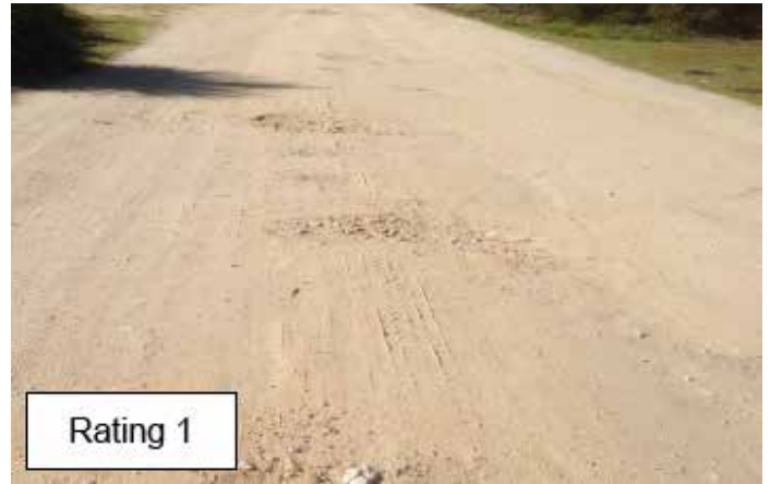
No evidence of protrusion
