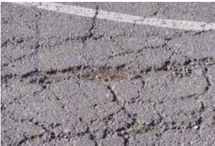
Localised cracking
