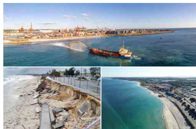
Top: Port Beach nourishment via rainbow dredging. Left: Coastal erosion at Port Beach. Right: Port Beach after sand nourishment completed © DPLH
